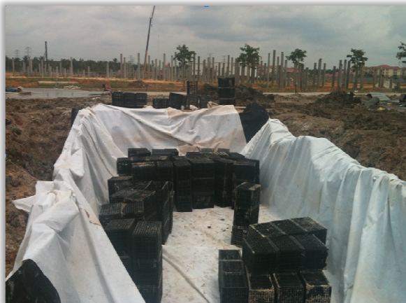
Cover EnviroModule into the pit
