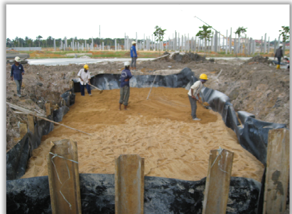
Back Filling with Sand at the top, followed by Top Soil
