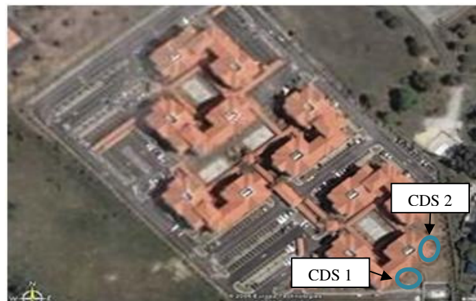
Figure 1. Location of Installed CDS at Amanah Apartment, UNITEN.
